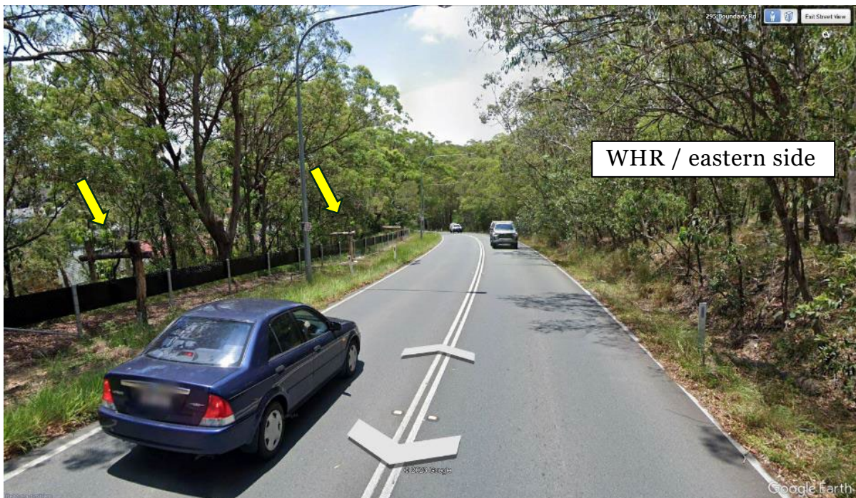
Figure 3. Image looking north-east along Boundary Rd where fauna exclusion fencing has only been installed on the non-reserve (western) side of the road. Numerous escape poles have been installed to provide koalas with an option to exit the road corridor (two examples indicated by yellow arrows).
